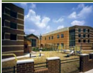
Port Towns Elementary School Bladensburg, MD
