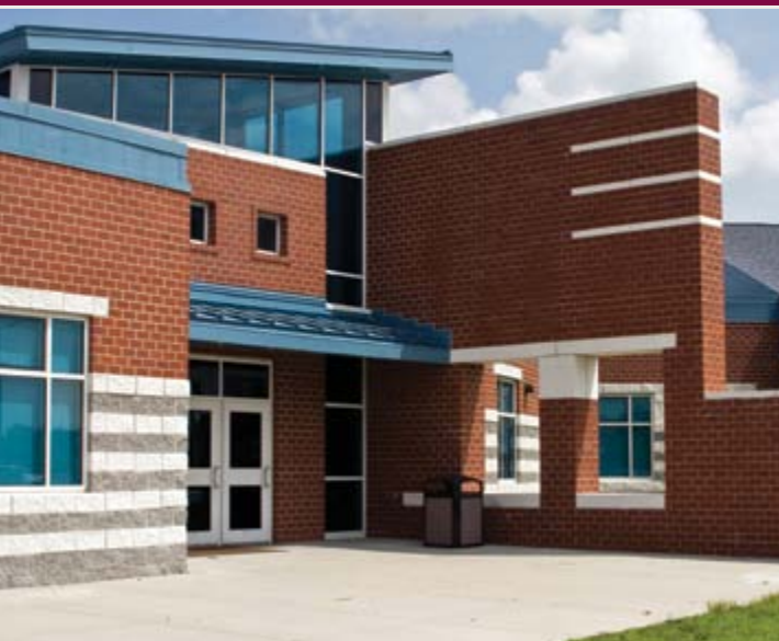
Creekside Elementary School - Suffolk, VA (left)
